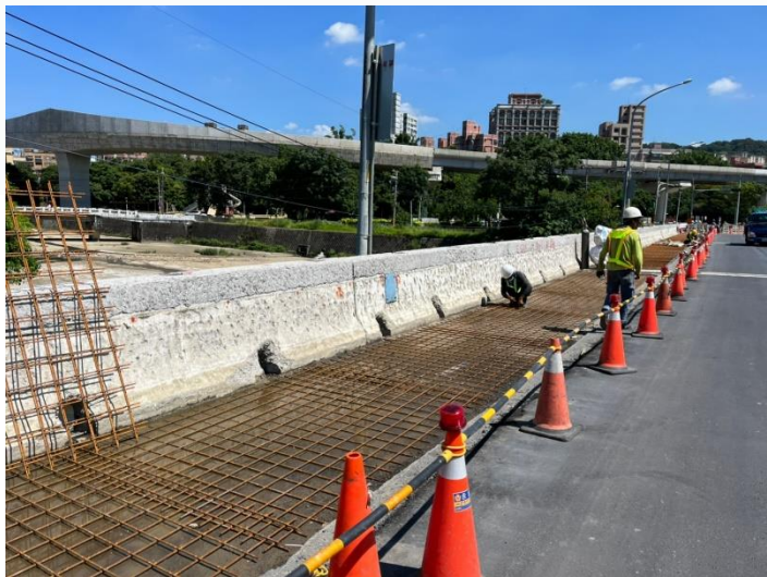
噴花地坪結構施作
